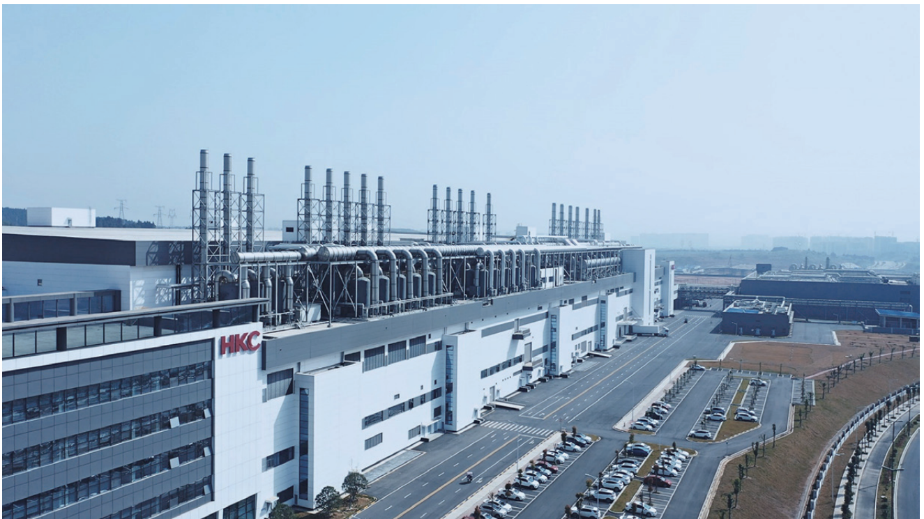
Huawei's UPS5000 empowers precision manufacturing
