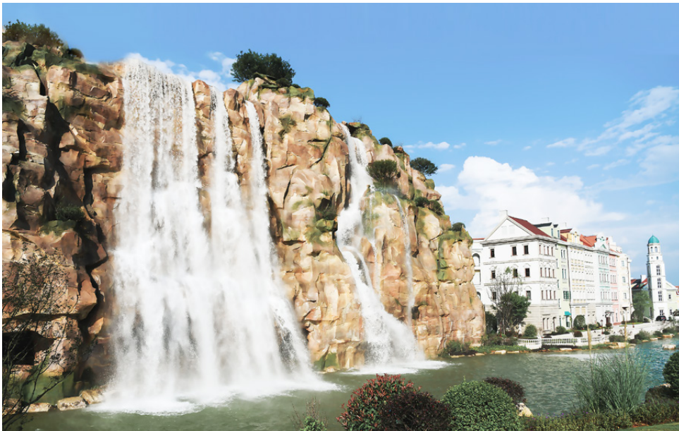
Huawei Cloud Gui'an data center
