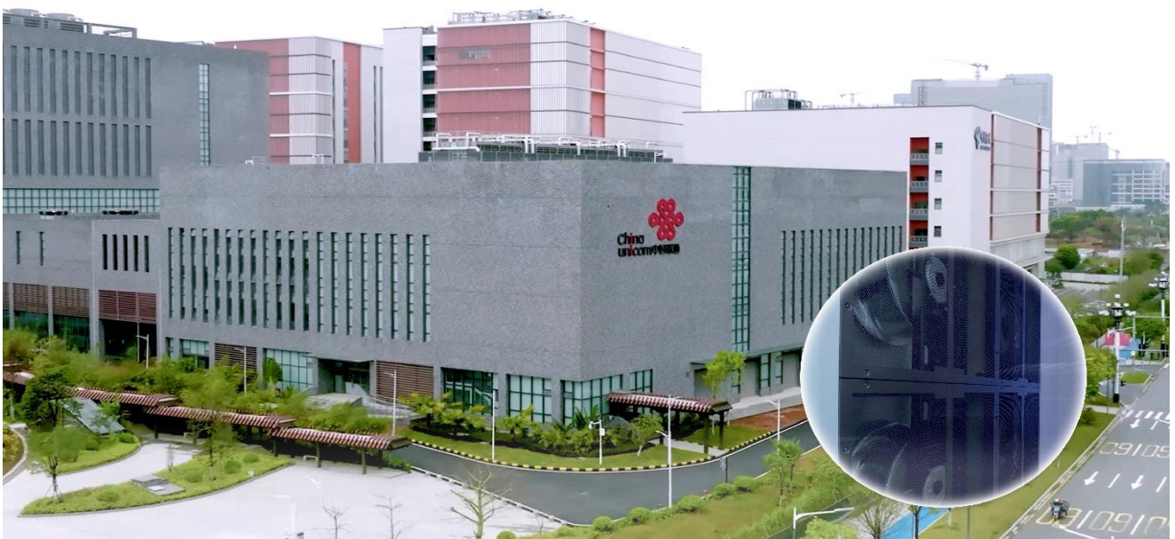
Huawei's Data Center Facility helps Guangzhou Unicom reconstruct energy-saving IDCs
